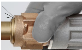
GG11: begin to unscrew combined unit - gas is released at screw connection.
