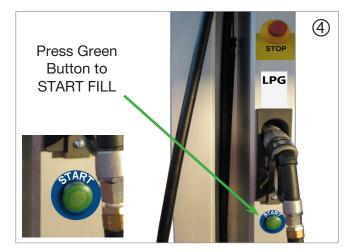
The nozzle is now safely attached to the fill point. You can leave the nozzle and press the green START button to commence refuelling.
